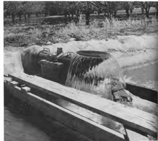
Pump outlets showing good flow of drainage water into ditch for reuse in irrigation as part of the Patterson drainage study.
