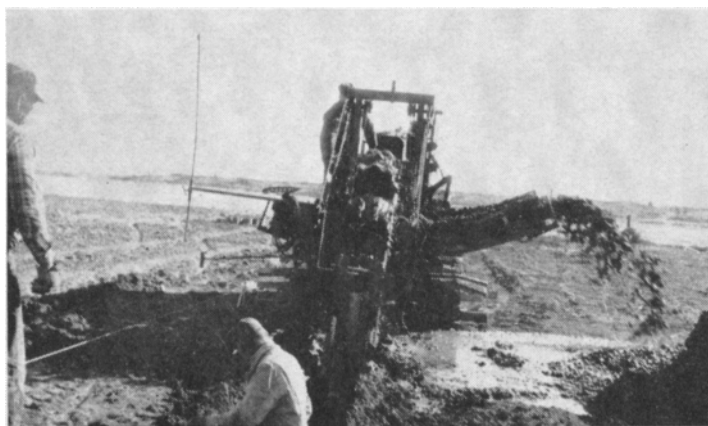
Drain trencher at work in Tulelake Basin.
