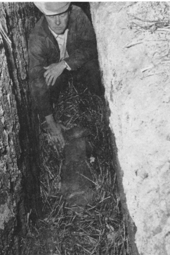
Straw envelope on 6 inch tile drain.
