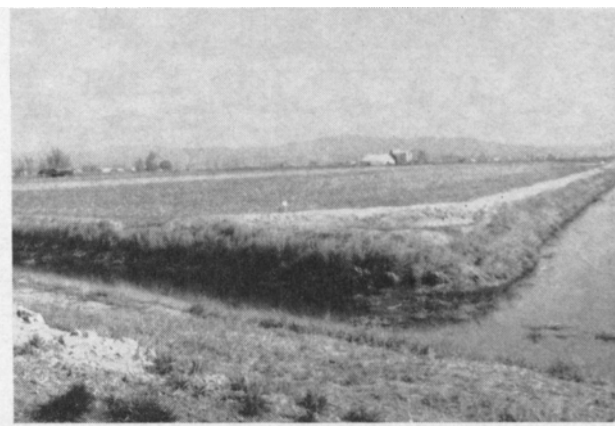
Open drainage system showing height of water in drains.
