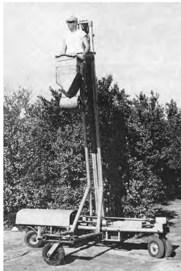
Principles of cylindrical coordinate system were used at Riverside in development of research prototype of commercial power ladder now in production.
