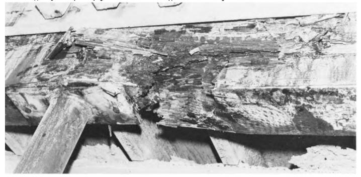
water entrapment. Untreated wood should not be on or near ground, because soil is a source of water and actively growing decay fungi. Design and construction details should direct rain water or condensation away from the structure. If wood must serve in soil or water contact, it should be pressure-treated with a preservative. These simple precautions may spare the building owner considerable repair costs.
