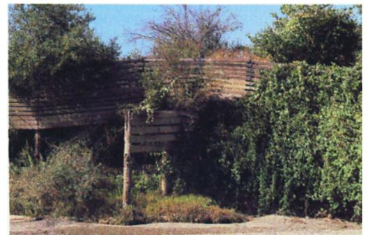
Wooden fences built along lower Dry Creek in earlier years effectively protected cut banks. They were often 3 to 6 meters tall, over 50 meters long, and constructed with large-dimension lumber.
