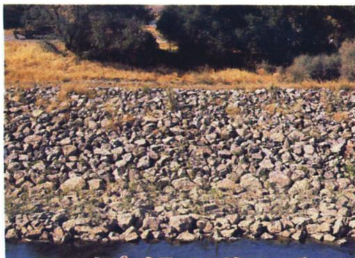
Riprapping with small rocks, used in a few areas along Dry Creek, requires a near paving of the banks with stones and leaves little space for sediment accumulation. We found no shrubs or trees established in any of the rock riprapped sites.
