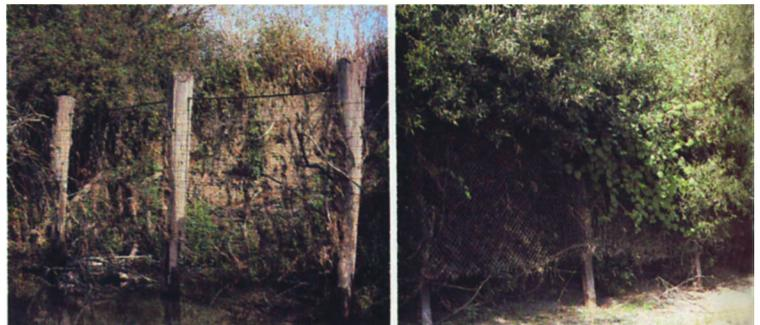
Hog-wire and chain-link fences at the base of cut banks reduce stream velocity and collect floating debris, further absorbing erosional energy. Seedlings become established at the base and lower slopes of cut banks behind the fences.
