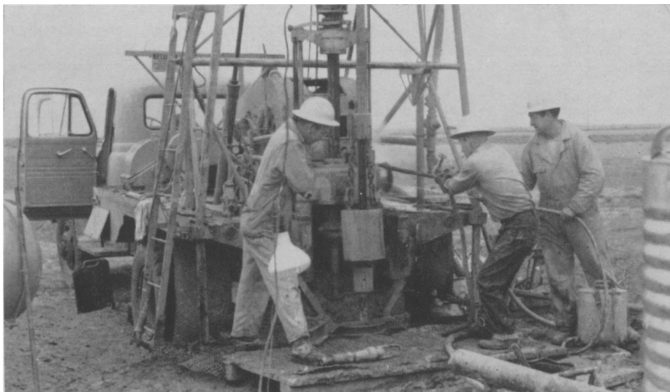
Fig. 3. Drilling for substrata core samples.
