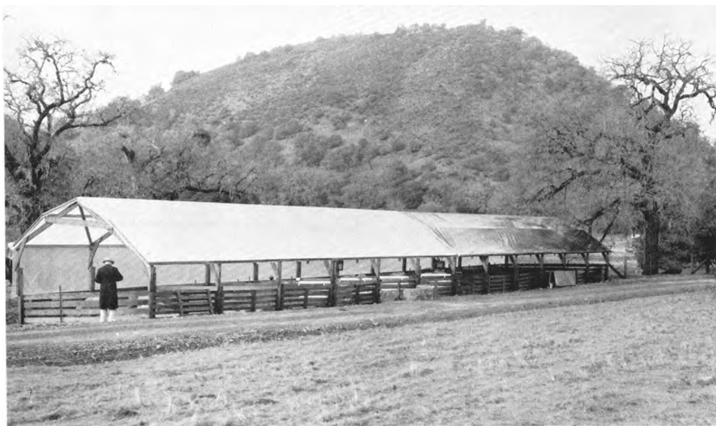
A 20' × 96' plastic-covered shelter. Shielded thermocouples for measuring air temperatures and globe thermometers for measuring spherical radiation were installed under the translucent film, under the black film, and outside the shelter.
