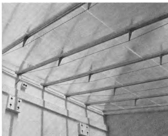
Double-pane plastic panels were used on roof and sides in latest phytotron modification at Davis, as seen in photo to left. Thin wire-stressed aluminum trusses, seen in photo below, were used to support plastic roof panels with minimum of light loss.
