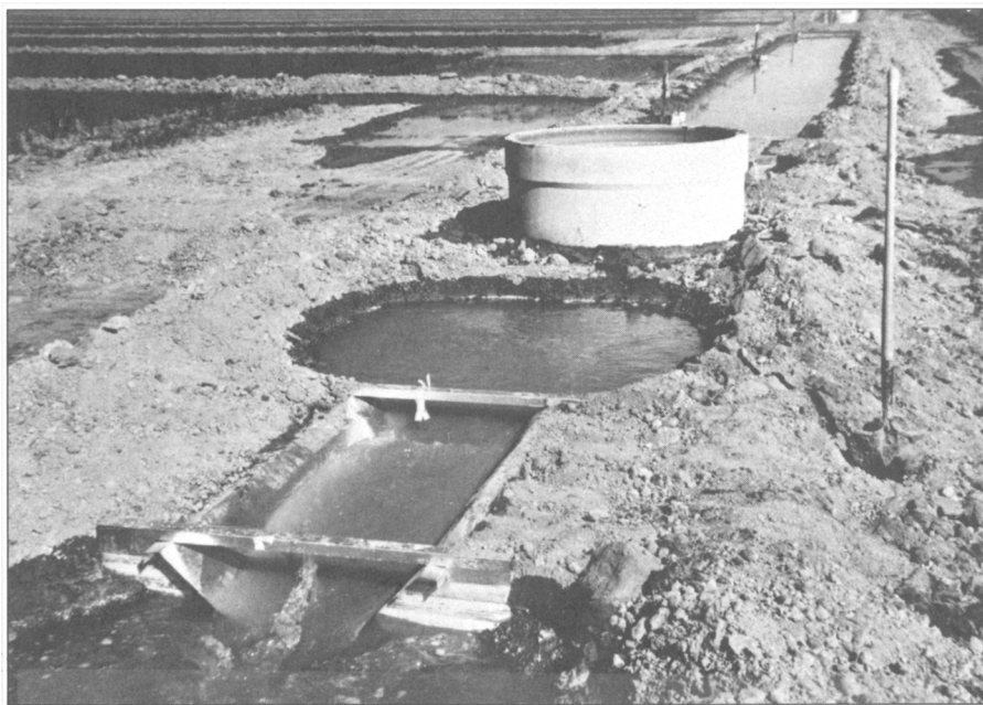
Fig. 3. Portable calibrated flume and two-way diversion chamber.
